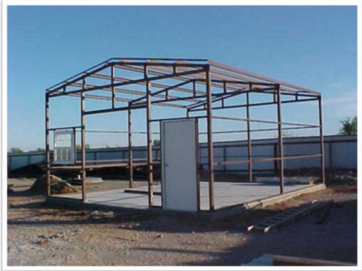
2. Steel Framing does not increase the fire load. Timber is combustible and there is at least 20kg of timber per square meter of floor area in a timber framed house. This is 75% of the design fire load of a houses content, which means that a timber framed house is carrying at least 1.75 times the fire load of a steel framed house. The higher the fire load, the more severe the fire.
